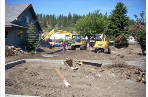
Special care was taken to preserve trees during site grading
